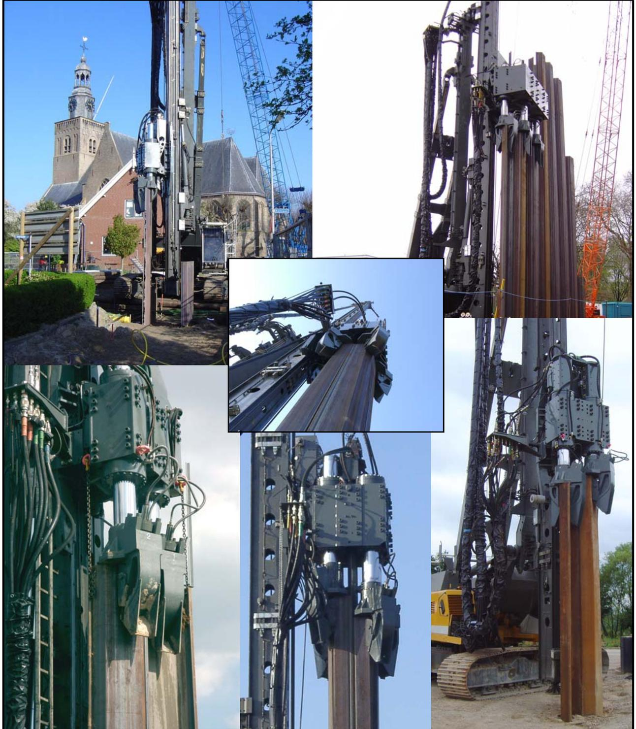
***Quiet, vibration-less installation and removal of steel sheet and foundation piles***
